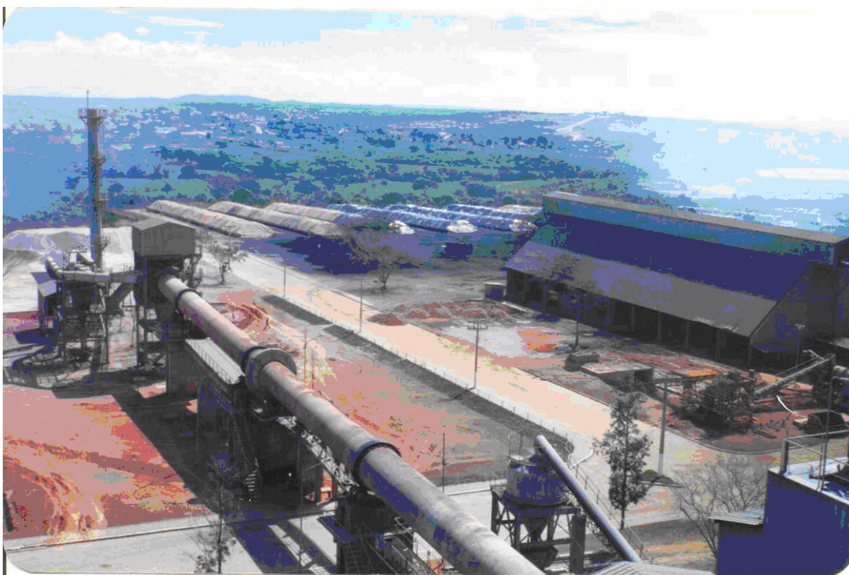
Figure 1 – Photograph of the plant, showing the dolomite kiln in the foreground and the piles of charcoal in the background
